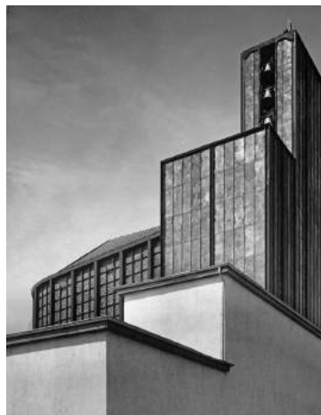
Otto Bartning Stahlkirche on the grounds of the International Press Exhibition (Pressa) , Cologne, 1928 Photo: Hugo Schmölz © Otto Bartning Archive TU Darmstadt
