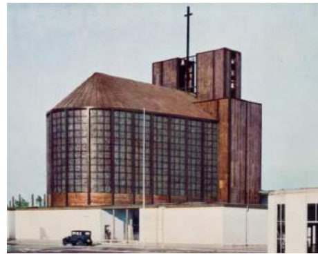
Otto Bartning Stahlkirche on the grounds of the International Press Exhibition (Pressa) , Cologne, 1928 Photo: Hugo Schmölz © Otto Bartning Archive TU Darmstadt
