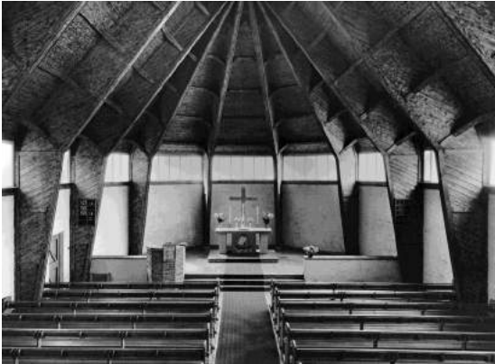
Otto Bartning Emergency church programme after 1946 Johanneskirche , Wuppertal-Elberfeld, 1948/49 Photo: Carl Schäfer © Archiv des Ev. Kirchenkreises Wuppertal
